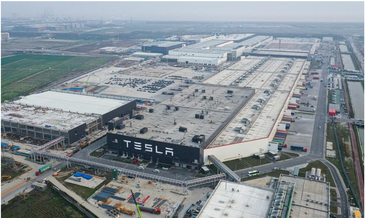
Fig. 3.1. Aerial view of Gigafactory Shanghai, April 2022. Source: [62]
